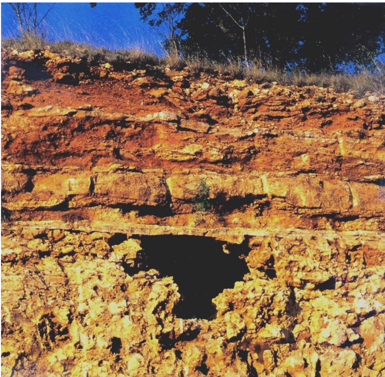
FIGURE 25. An example of a cavity dissolved in limestone (the Edwards Limestone) in central Texas. Note that the roof of the cavity, which is about a meter across, has not yet collapsed.
