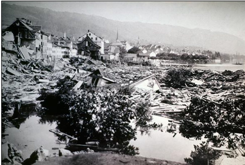
FIGURE 23. Town of Zug after the 1887 catastrophe.
